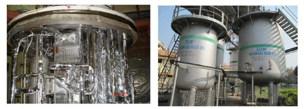
Figure 2: Internal view of the cold box of Helium Refrigerator 1
