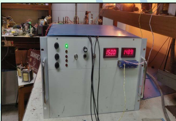
Figure 2: Power supply components assembled within 19inch cabinet
