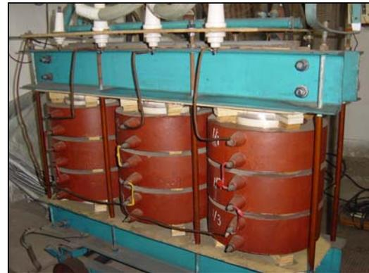
*High voltage resin-cast water-cooled transformer for Final Amplifier Power Supply (FAPS) of room temperature cyclotron*
