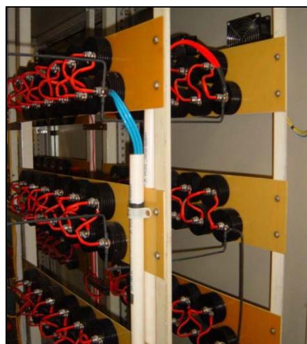
*Rectifier bank assembly for anode power supply*
