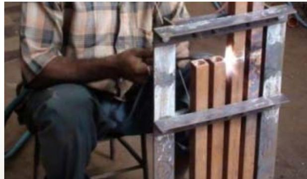
Figure 2: Brazing joint of conductors being done with 12mm gap keeping similar to actual situation.
