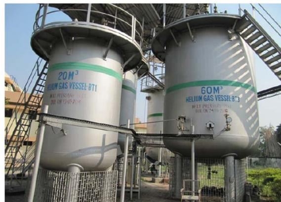
Figure 3 Buffer Tanks as storage of pure helium gas
