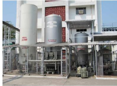
Figure 5 Liquid Nitrogen Tanks for storage and delivery of LN<sub>2</sub>
