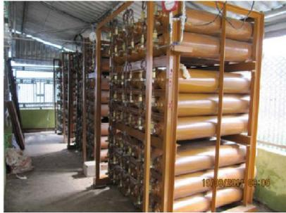
Figure 4 Three Quads for Impure bank
