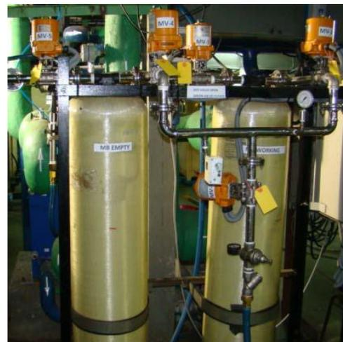
Fig. 6: PLC based automatic Mixed Bed unit
